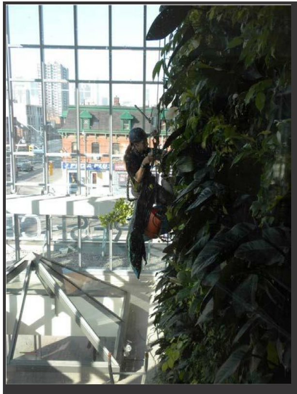
Although much of the maintenance of the Living Walls can be considered 'routine', there are times when the maintenance occurs 20 metres off the ground
